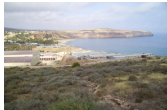
Souk Tleta Desalination plant Location: Souk Tleta-Tlemcen (Algeria) Capacity: 200.000 m 3 /day
