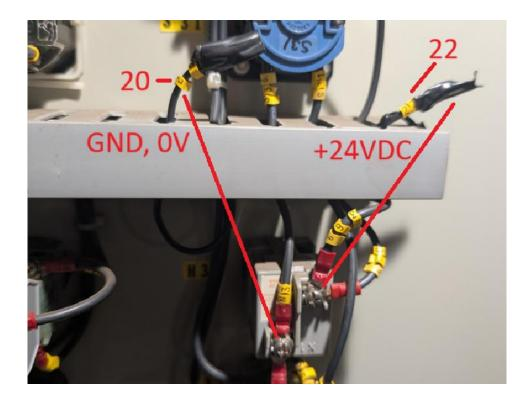
These two wires I can't see in any of the documentation, and they've been added in some rebuild, cable shoes, cable type and pathing are all nonstandard to the switchboard. While these were connected fuse F303 instantly blows. I have no idea when or why there are added, cables disconnected for now. After resetting breaker, axel generator breaker automatically syncs to switchboard again and status lights works as they should
